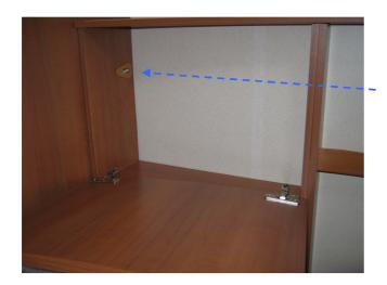
The bottom part of the cupboard in the wash room is divided into segments, that makes the disassembly of the toilet easier. Unscrew the left cabinet element and take it out completely.
