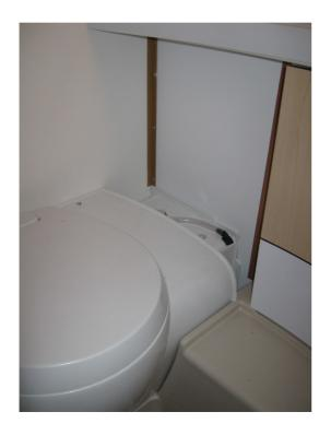
After the element of the cupboard has been taken out, the bottom of the cloakroom wall should be pulled out carefully. This is necessary to prevent that the toilet will damage the stop bar of the cloakroom wall. The toilet can now be raised and removed from the washroom.
