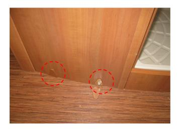
First step is to unscrew the lower connections at the cloakroom wall because you have to pull out the wall later on .
